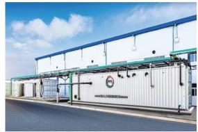
Inlet:CODCr < 2000mg/L,TDS≈28000mg/L Permeate:CODCr ≤70mg/L,TDS≤800mg/L Capacity:1000m<sup>3</sup>/d(Phase I)1000m<sup>3</sup>/d(Phase II)
